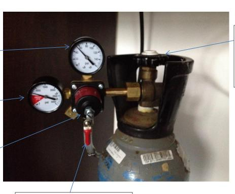
Red/Brass Lever in Vertical Position – Tank TURNED ON C02 Tank Main Valve Handle – Turn Completely Clockwise for tank to be OPEN
